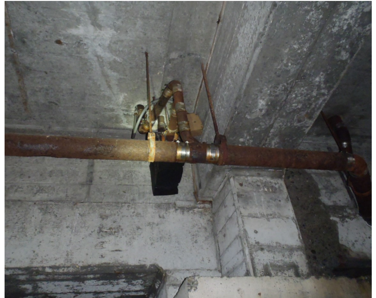
Corroded Sewer Lines and Hangers
