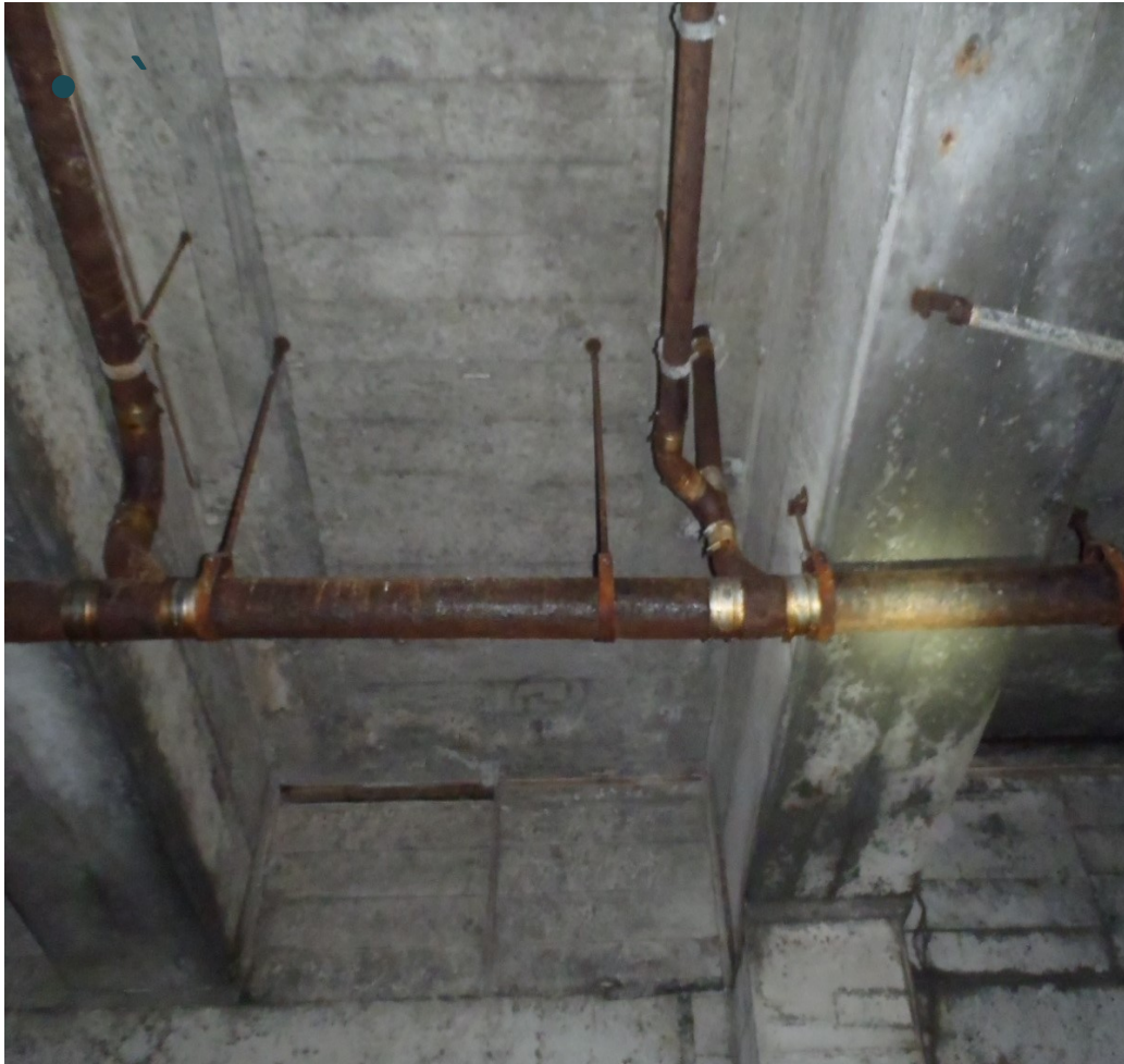
Corroded Sewer Lines and Hangers
